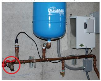
NOTE: Try to use as low of a valve as you can which will allow more of the system to be drained and reduce the amount of water that will leak when the transducer is removed from the piping.
