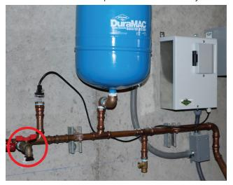
NOTE: Try to use as low of a valve as you can which will allow more of the system to be drained and reduce the amount of water that will leak when the pressure switch is removed from the piping.
